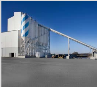
Tower plant with 2 – 6000 litres mixers for production of ready-mix concrete.
