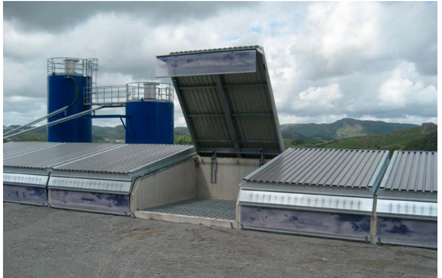
Bins placed in the ground with hydraulic operated cover.
