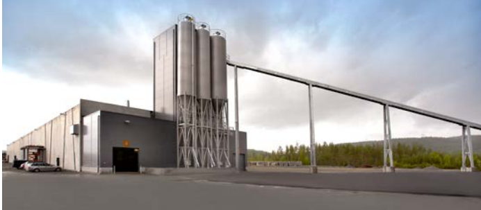
Tower plant with 2 – 2250 litres mixers for production of railway sleepers.
