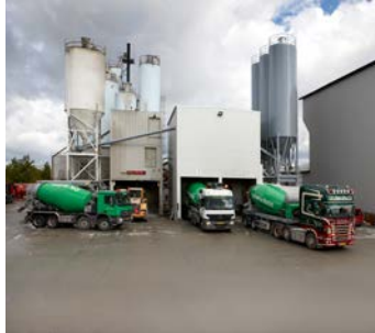
Modernisation of existing ready-mix concrete plant with a Haarup 6000 litre mixer.
