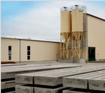
Concrete slats factory with complete Haarup batching and mixing plant.
