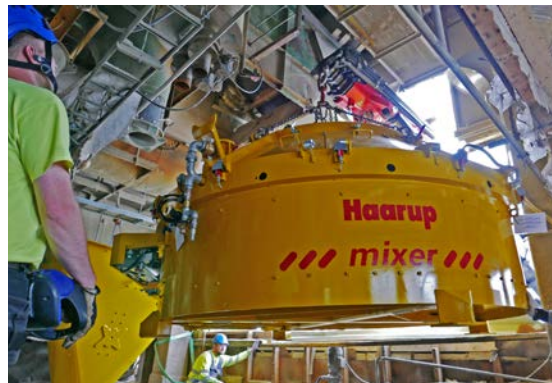
Modernisation of plant with new Haarup 3000 litre mixer.
