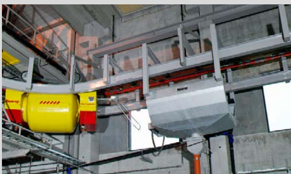
Washing station for cleaning of 2000 litre duo-speed concrete travelling bucket.
